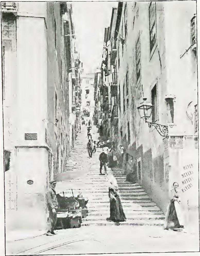
THE THRESHOLD OF OLD LISBON
